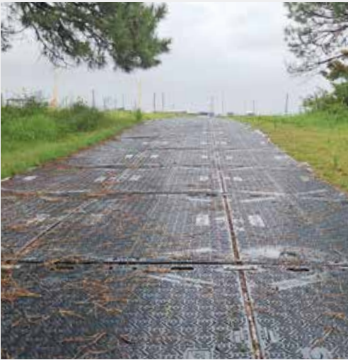
Truck access route Pinned mats created a defined route for loaded waste truck movements across grassed land.
