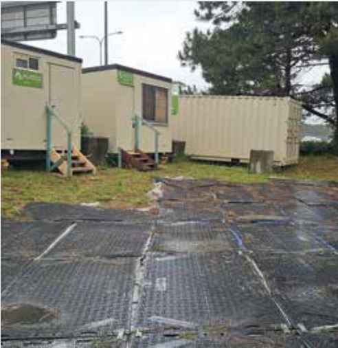
Compound areas Mats were underlaid with geofabric & polyethylene sheeting for maximum environmental protection.
